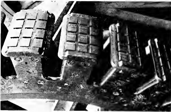
FIG. 17—GRID DAMPERS ON FIELD POLES
